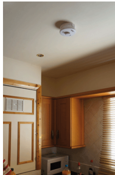
The London Student Group has already installed heat and smoke alarms in its properties.
